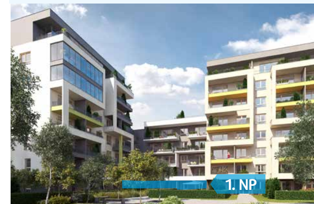
Pohled na dům z vnitrobloku / Building View From the Courtyard
