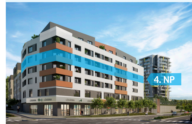
Pohled na dům / Building View
