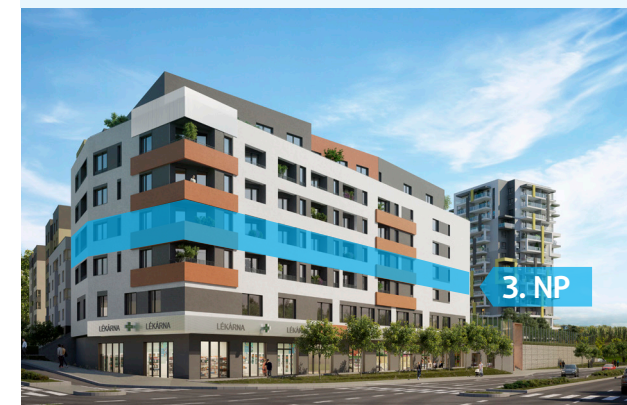
Pohled na dům / Building View
