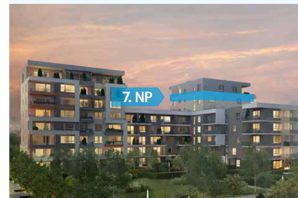
Pohled na dům z vnitrobloku / Building View From the Courtyard
