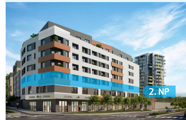
Pohled na dům / Building View
