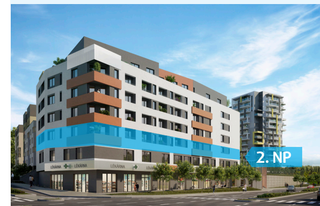
Pohled na dům / Building View
