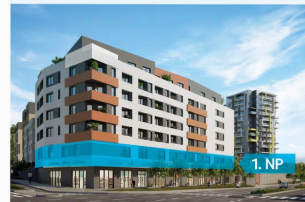
Pohled na dům / Building View
